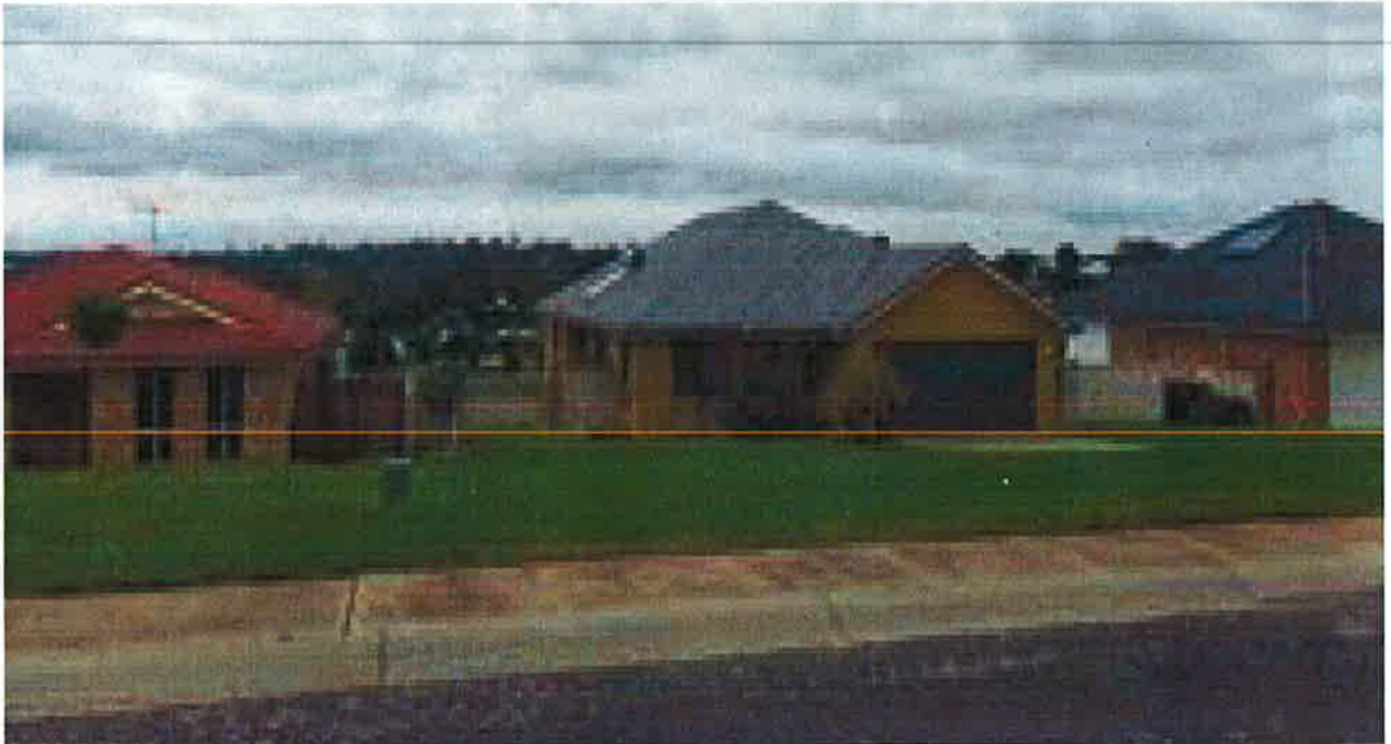
Figure 6 - Site photo – 10 William Street, Molong
